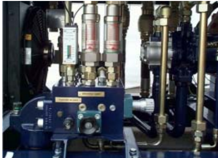
VISCOTHERM Control Block
